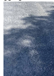
Compacted mineral sub-base
